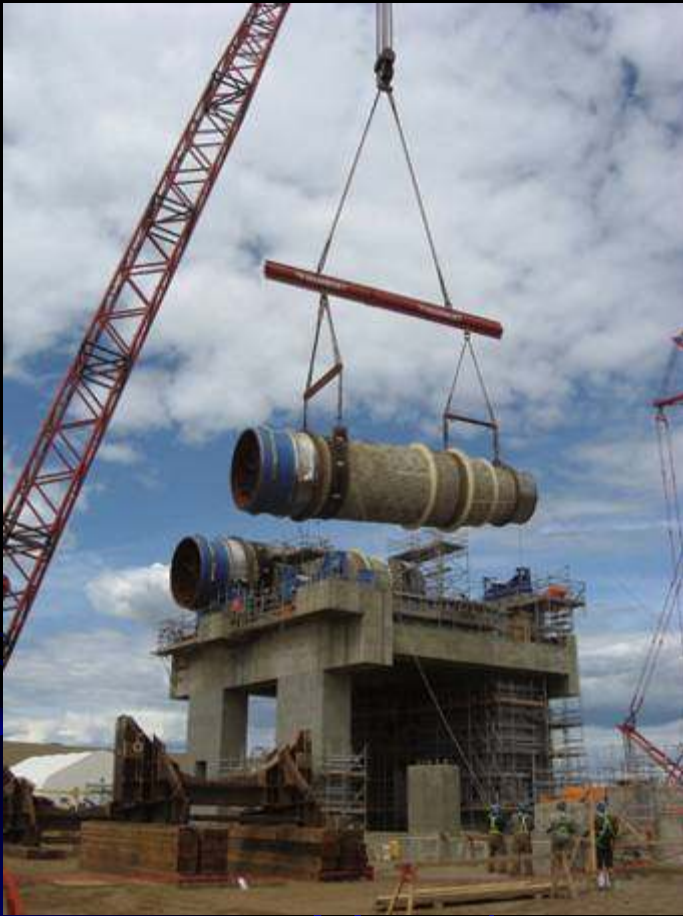
Heavy lift of rotary crusher at C&C silo
