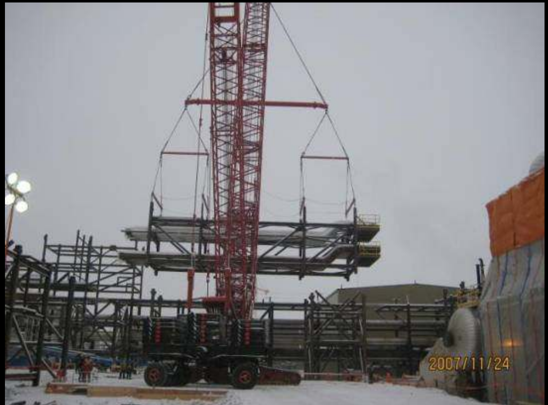
First pipe module being set at U&O silo
