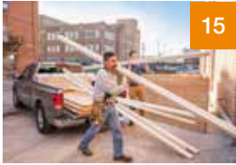
Construction's productivity problem
