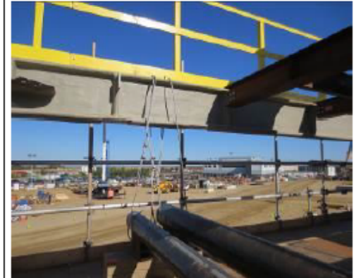
Figure 4: Two pipes that have been temporarily secured with wire ropes and clamps (lashing).
