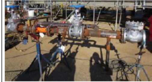
Figure 2: A smaller pipe system that is being assembled while sitting on two pipe stands (one on each end). Note the various valves being used in this system.
