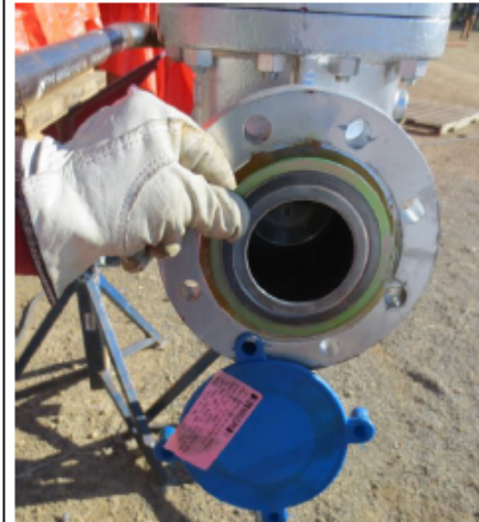
Figure 3: A valve with casket that will be secured once the next spool in the system is connected.
